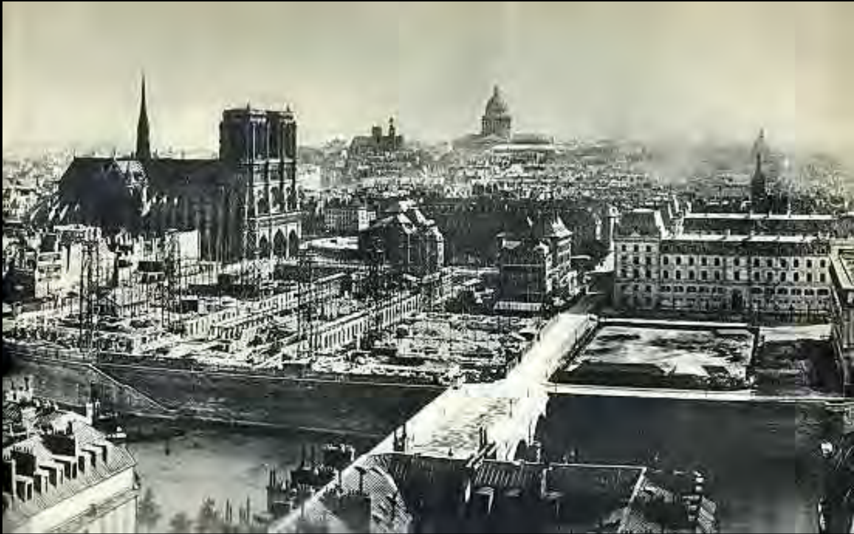
Notre Dame and Ile de la Citie during demolition of the buildings near the cathedral.
