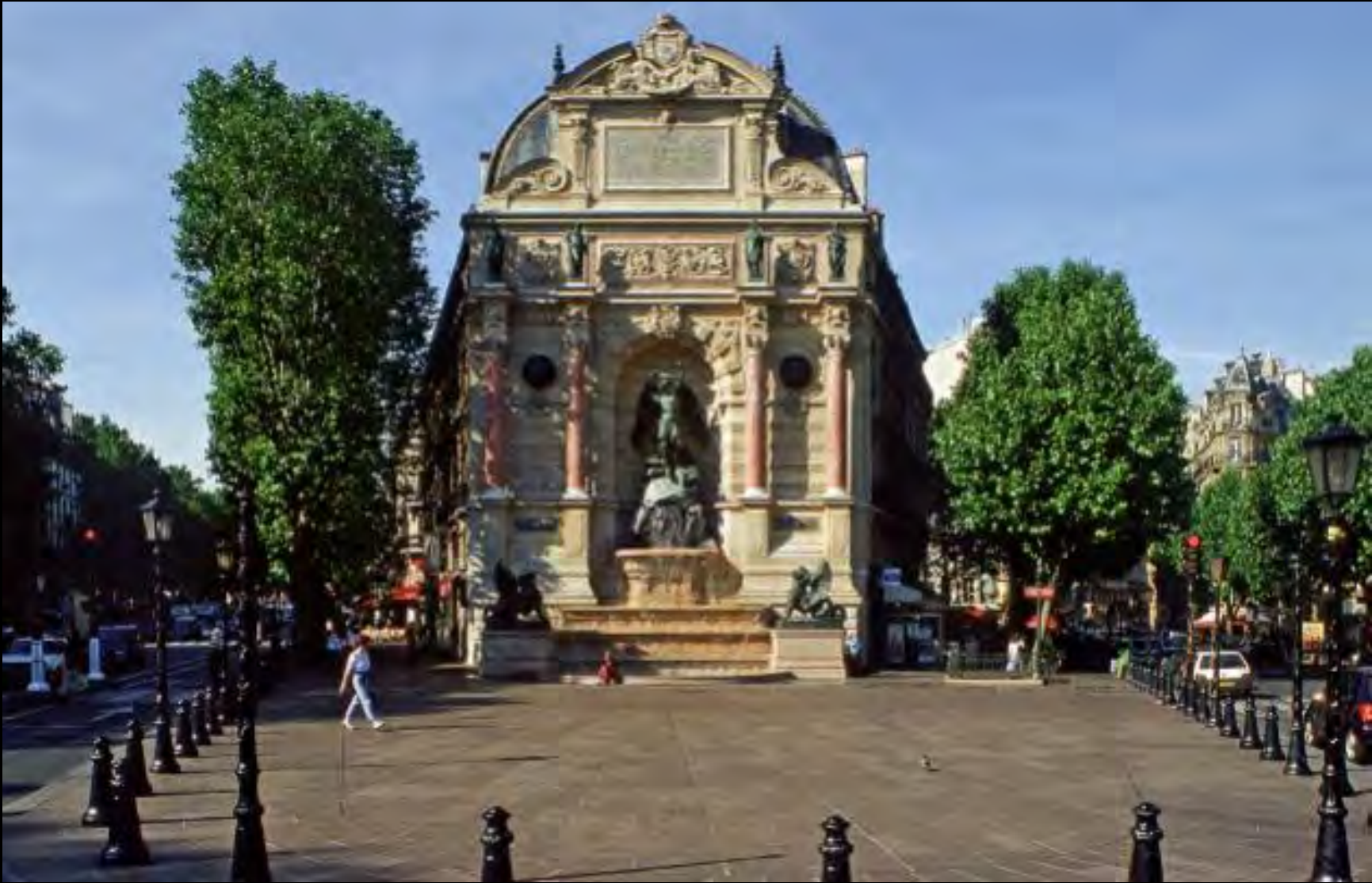
The Fontaine Saint-Michel (1858–1860), designed by Gabriel Davioud, marks the beginning of Boulevard Saint-Michel.
