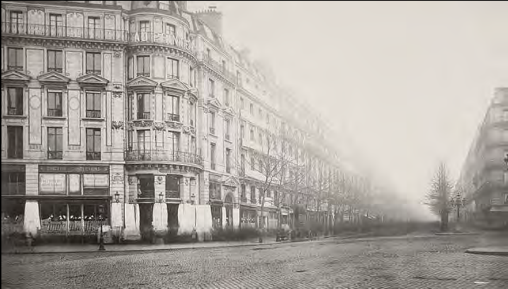
Newly completed Boulevard Haussman with landscaping, and new buildings, including the Au Printemps Department store.
