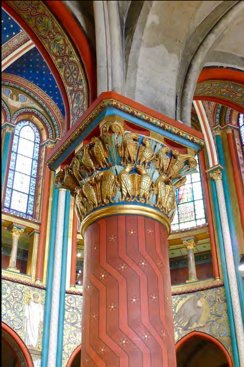
Column capital after restoration.
